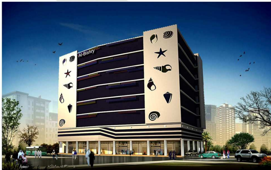
Al Bishry Project (G2) Status: ongoing
